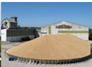
TEMPSTOR Temporary storage 5200 m3 Auger loading
