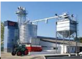
STORAGE : CEREALS DRYING Hopper bin + building Dryer Fixed loading Unloading Bulk loading bin
