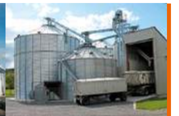
STORAGE : CEREALS DRYING Silos X4 Drying bin Loading and unloading Dust extractor
