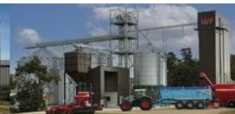
STORAGE : CEREALS DRYING Silos X2 Hopper bin Energy saving Dryer
