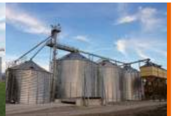
STORAGE : CEREALS DRYING Silos X4 Drying bin Fixed loading Unloading
