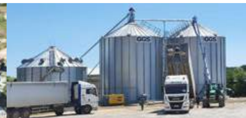
STORAGE : CEREALS Slovakia Drying bin Silos X2 Mobile auger
