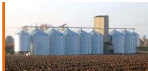
STORAGE : CEREALS Hopper silos X2 Flat bottom silos X5 Fixed loading and unloading
